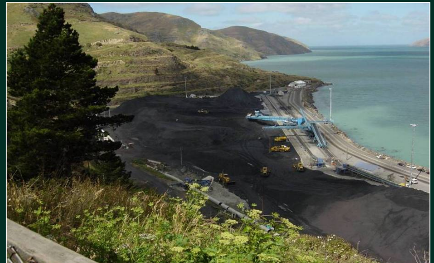
Port Lyttelton coal stockpile and handling facility
