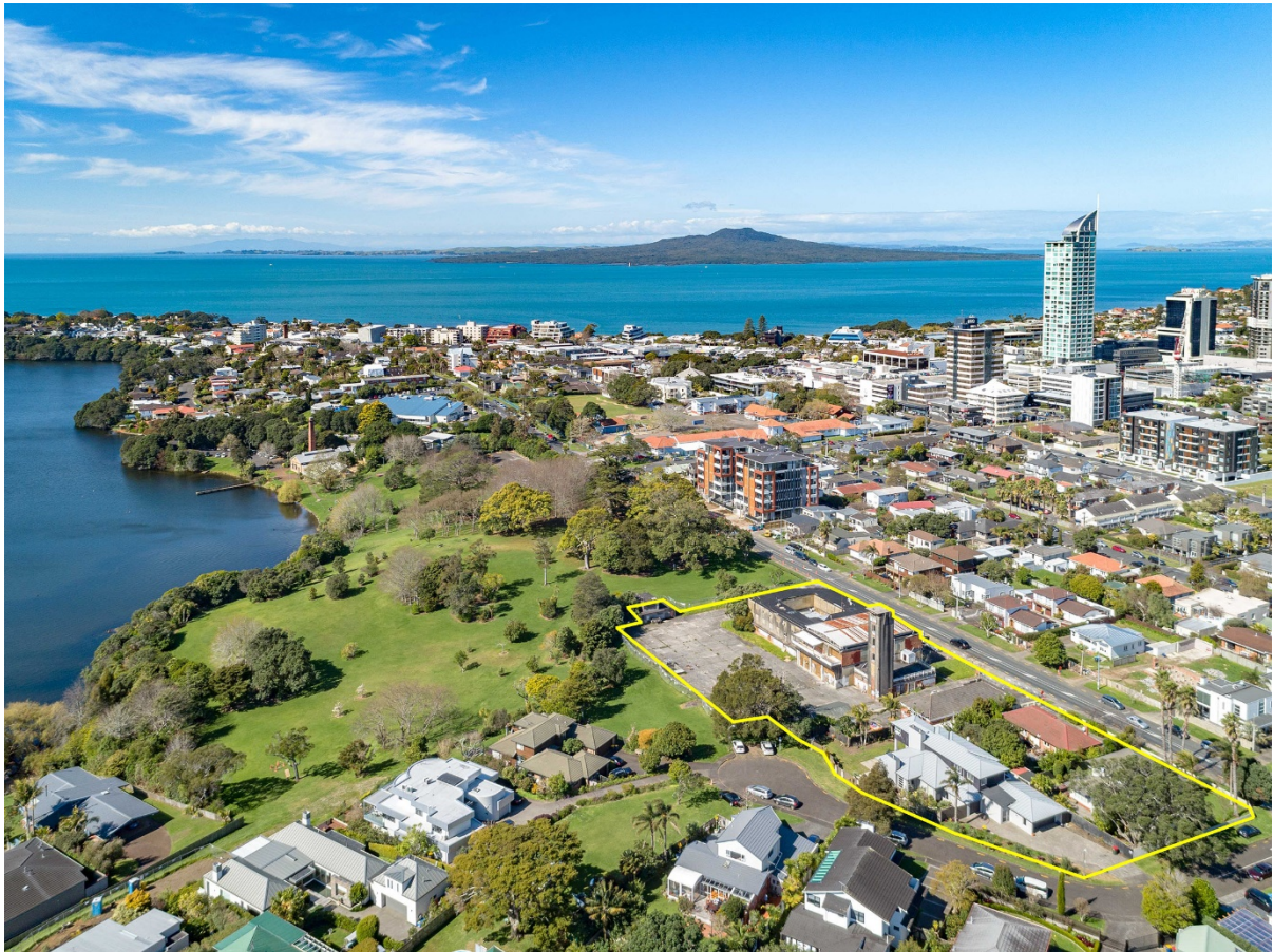
Aerial photo of Ryman's new Takapuna site.
